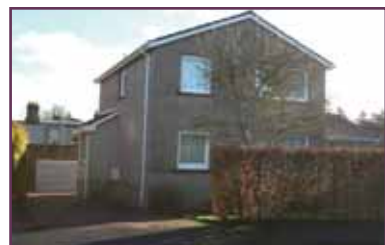
2 Barrcraig, Bridge of Weir OFFERS OVER £280,000
