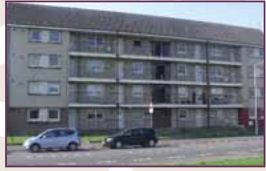
69 Springbank Road, Paisley
